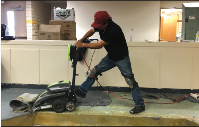
Lorenzo Rios removes old carpet in preparation for installing new carpet tiles in Oro Grande's library.
