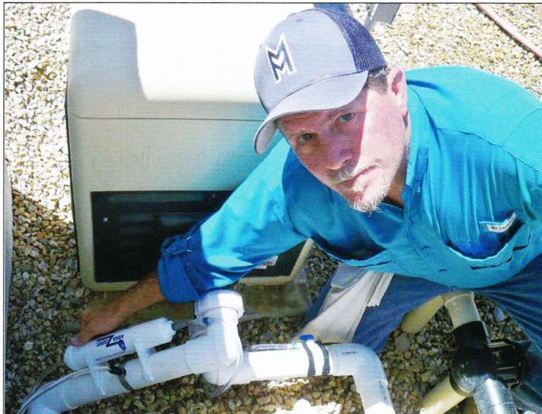
Dennis Kentch, of D & J's Pool & Spa Service & Repair, invented a device that uses pool water to irrigate landscaping while keeping the pool water at the desired chemical balance.
